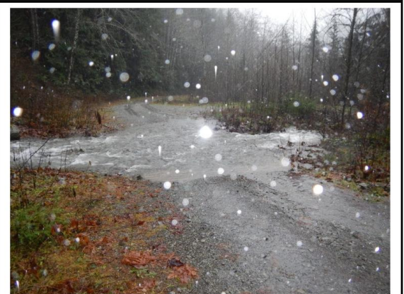
Road 2060: rock ford on seasonal stream; more dip in road needed to keep in channel
